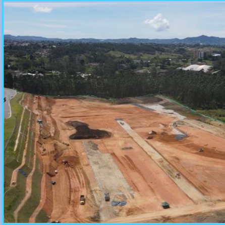
New factory in Colombia
