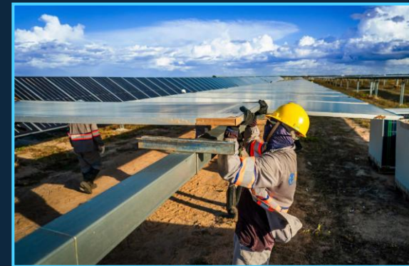
ELECTROMECHANICAL AND CIVIL INSTALLATION
