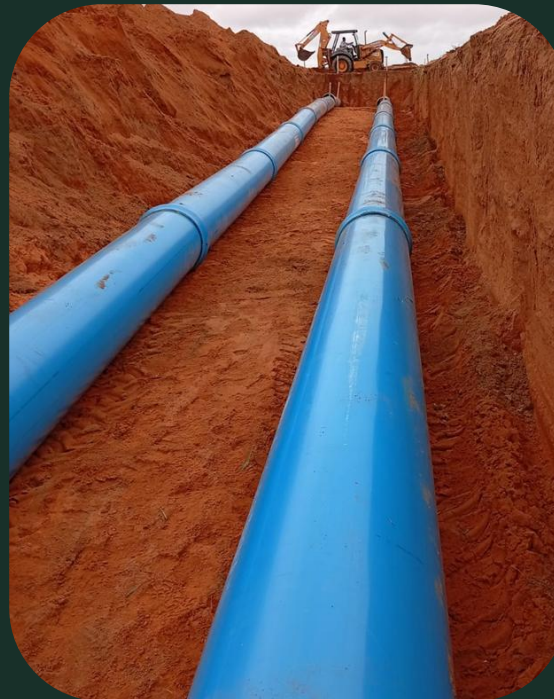
Water Main Installation 500mm
