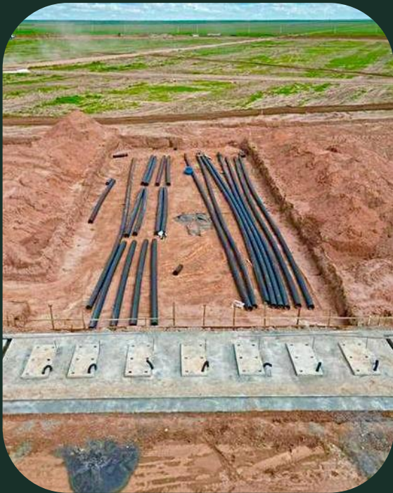
Construction of the pump house
