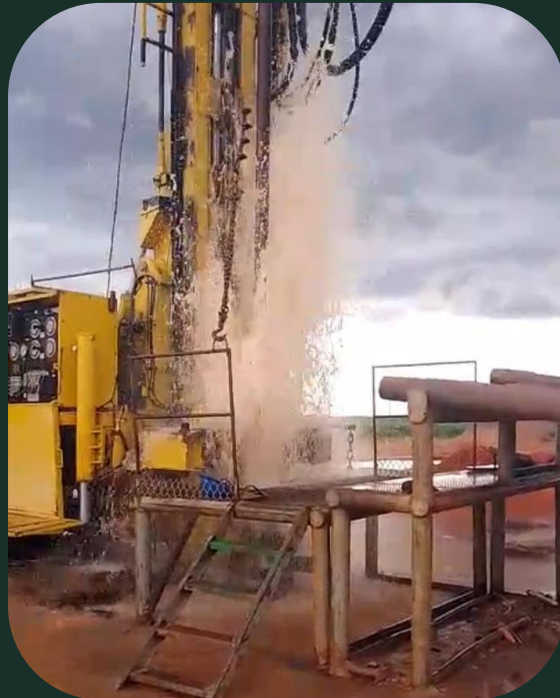
Well drilling 300m 3
