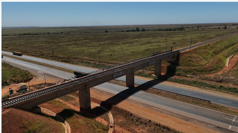
Km 8 – Viaduct over BR163
