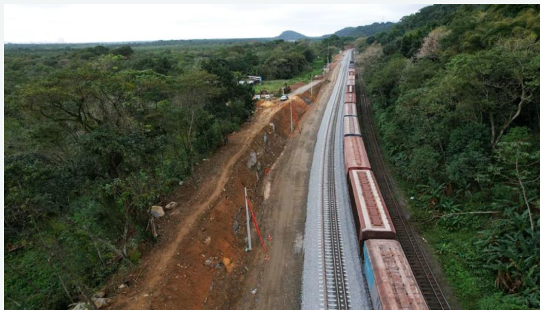
Sidings extensions | Paratinga Fase 1 - km111+453
