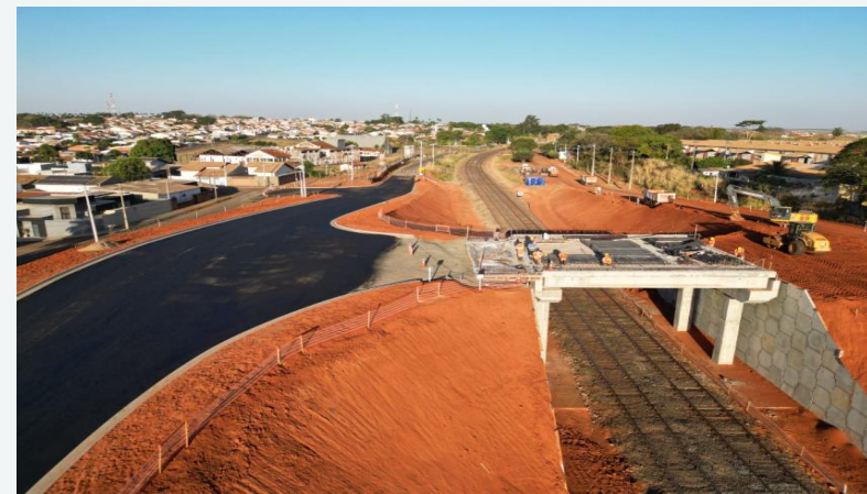
Road Overpass | Fernandópolis - km339+930
