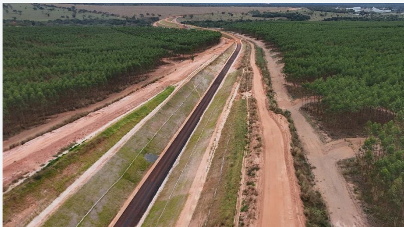
Km 25 – Platform concluded
