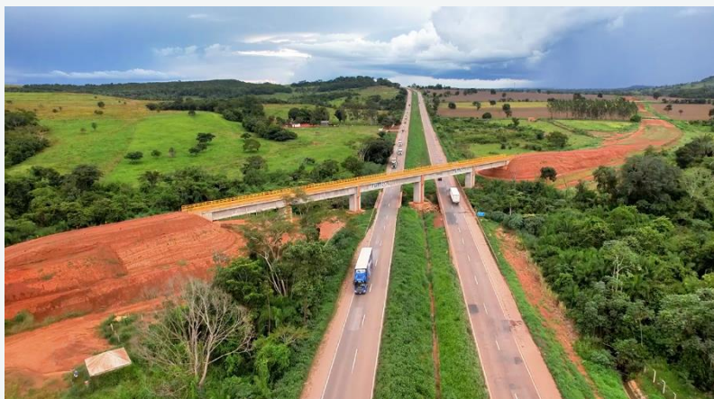
Km 72 – Bridge over the “Rio Tugore”
