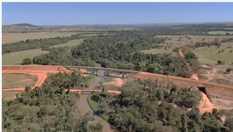
Km 87 – Bridge over the “Rio Areal”
