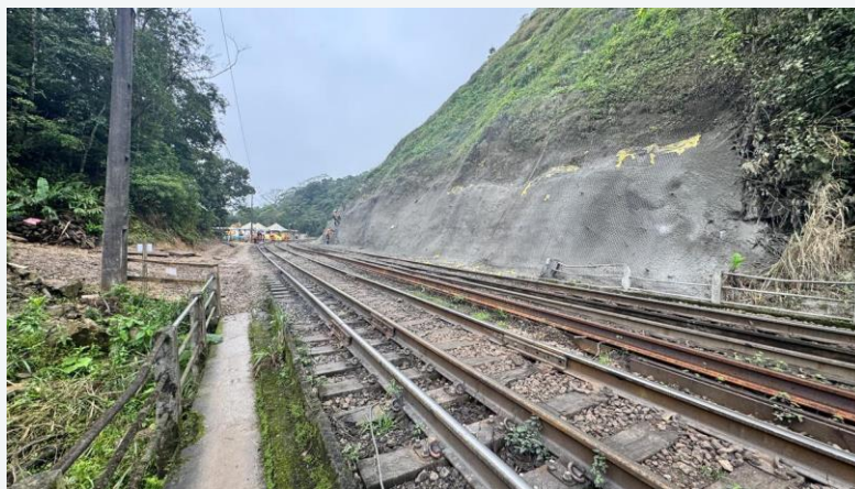
Slope Stabilization Works | Km 79 e 80
