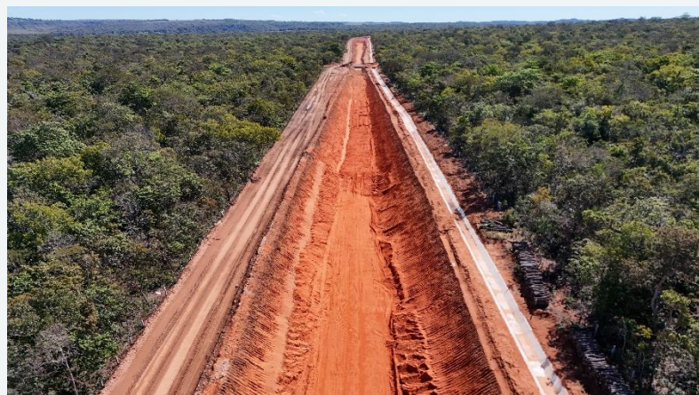
Km 133 – Drainage channels completed and ongoing earthworks
