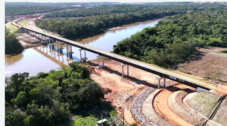
Km 35 – Bridge over the “Rio Vermelho”
