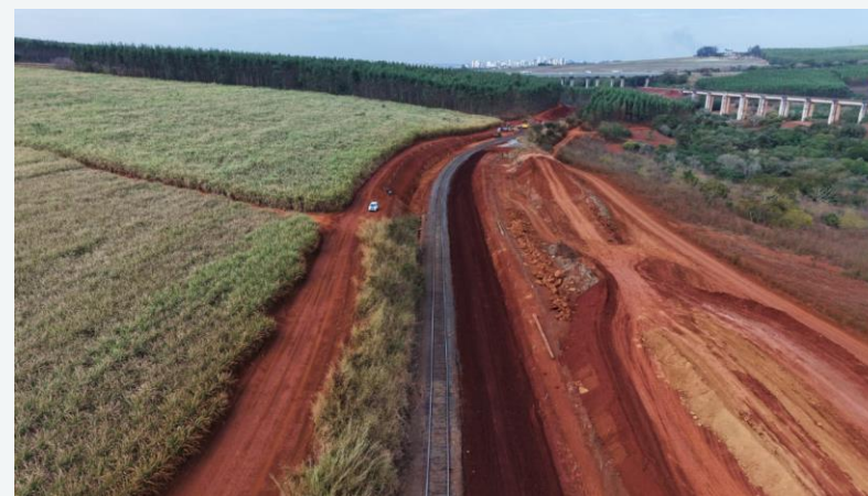
Railway Line duplication | Limeira - km109+352
