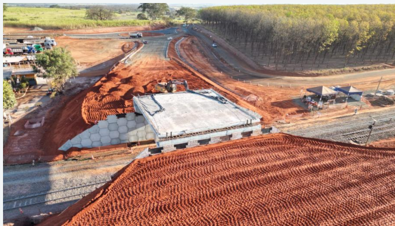
Road Overpass | Fernandópolis - km342+460
