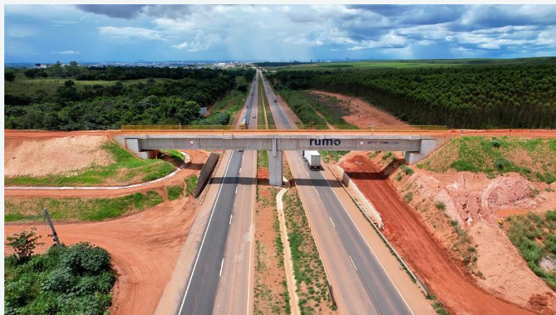
Km 26 – Viaduct over BR163
