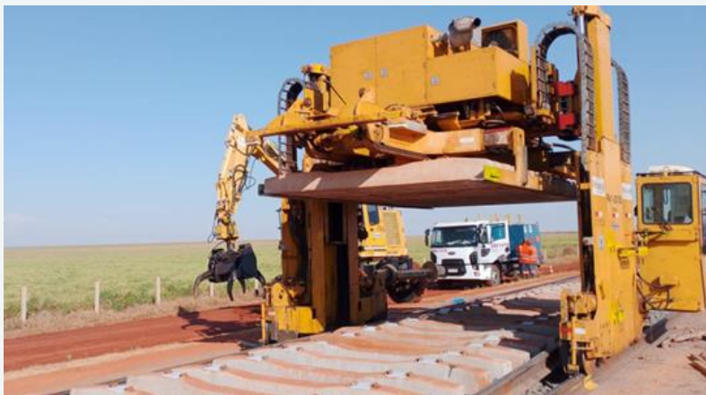
Km 10 – Portal Structure
