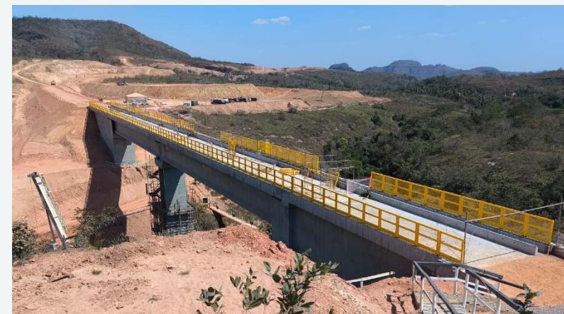
Km 113 - Bridge over the “Rio São Paulo”
