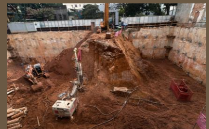
Excavation and ground anchors
