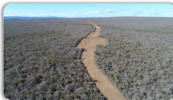
Earthmoving at the Campo Largo II Wind Complex
